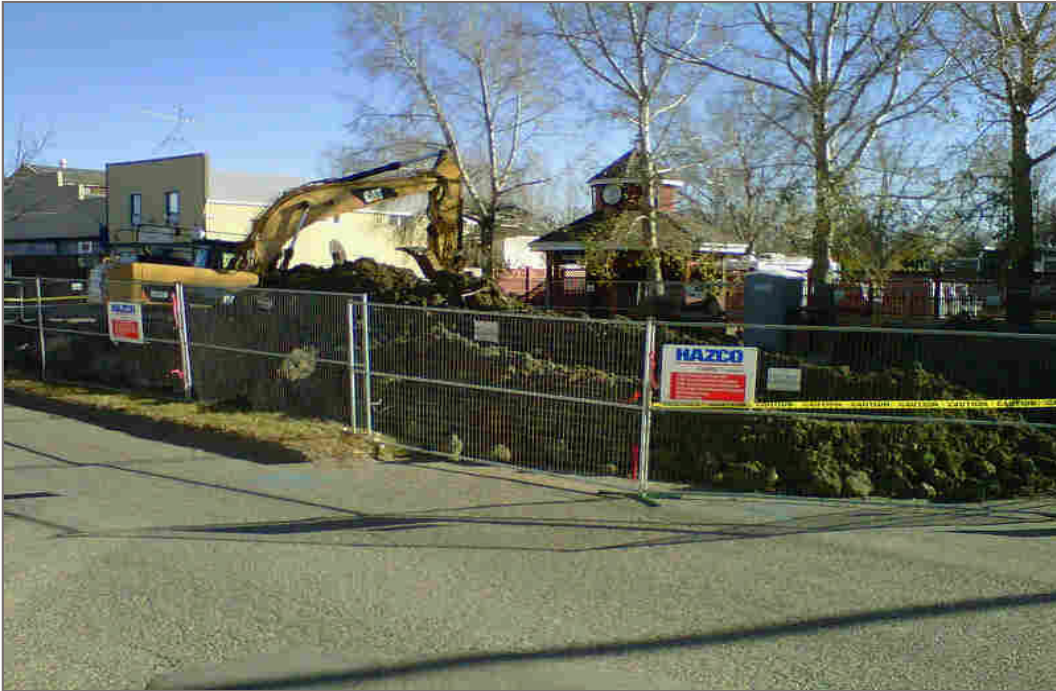
Photo 1: View looking south at trackhoe excavating tank nest.
