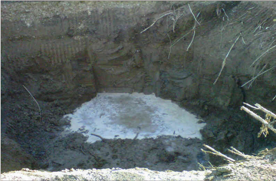
Photo 7: View looking east at excavation, showing groundwater infiltration.
