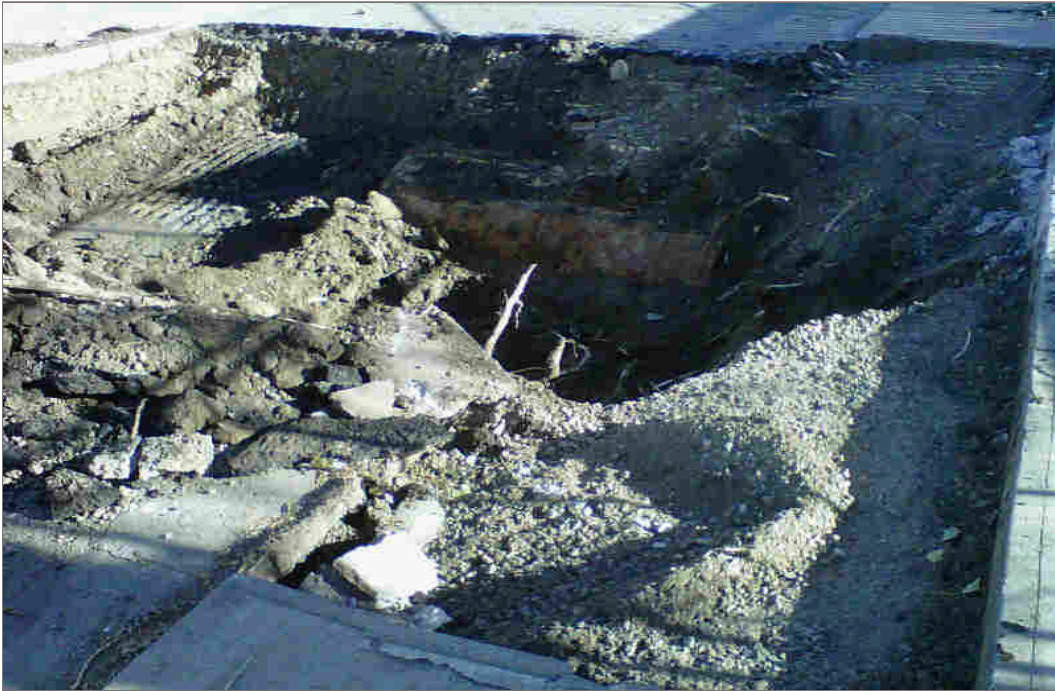
Photo 5: View looking east at underground storage tank within the excavation.
