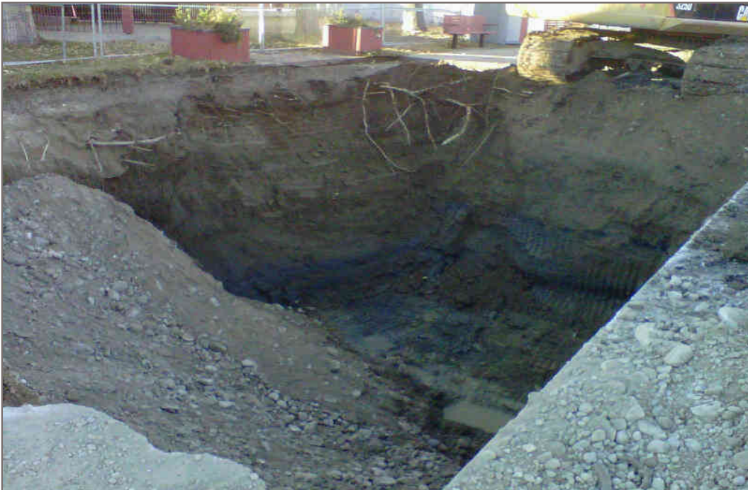
Photo 8: View looking southwest at excavation. Note fill material on left hand side of photograph to stabilize east wall.
