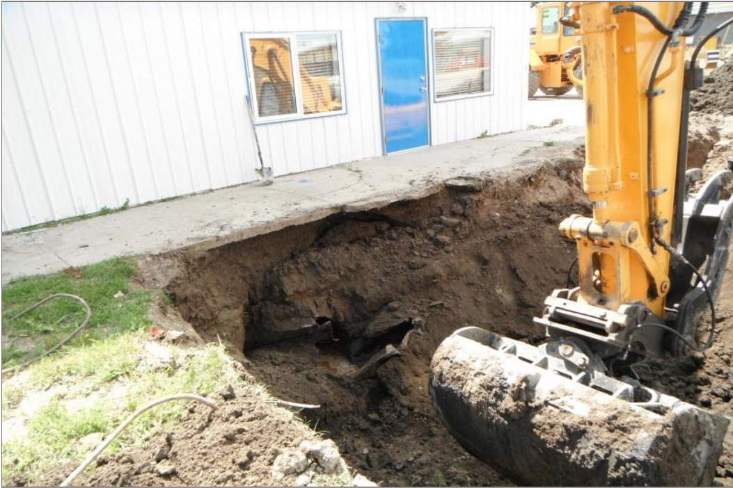
Photo 3: View of southeast corner of excavation and location of USTs.
