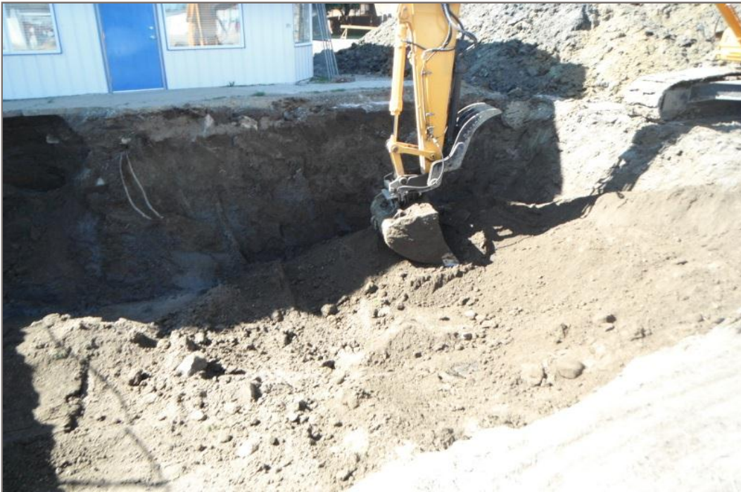
Photo 6: View looking southwest at the excavation limits. Note the piping and void where the USTs were removed in the left hand side of the photograph.
