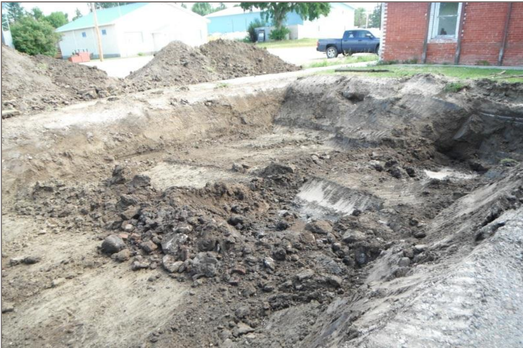
Photo 2: View looking northeast at excavation with non-impacted material removed.
