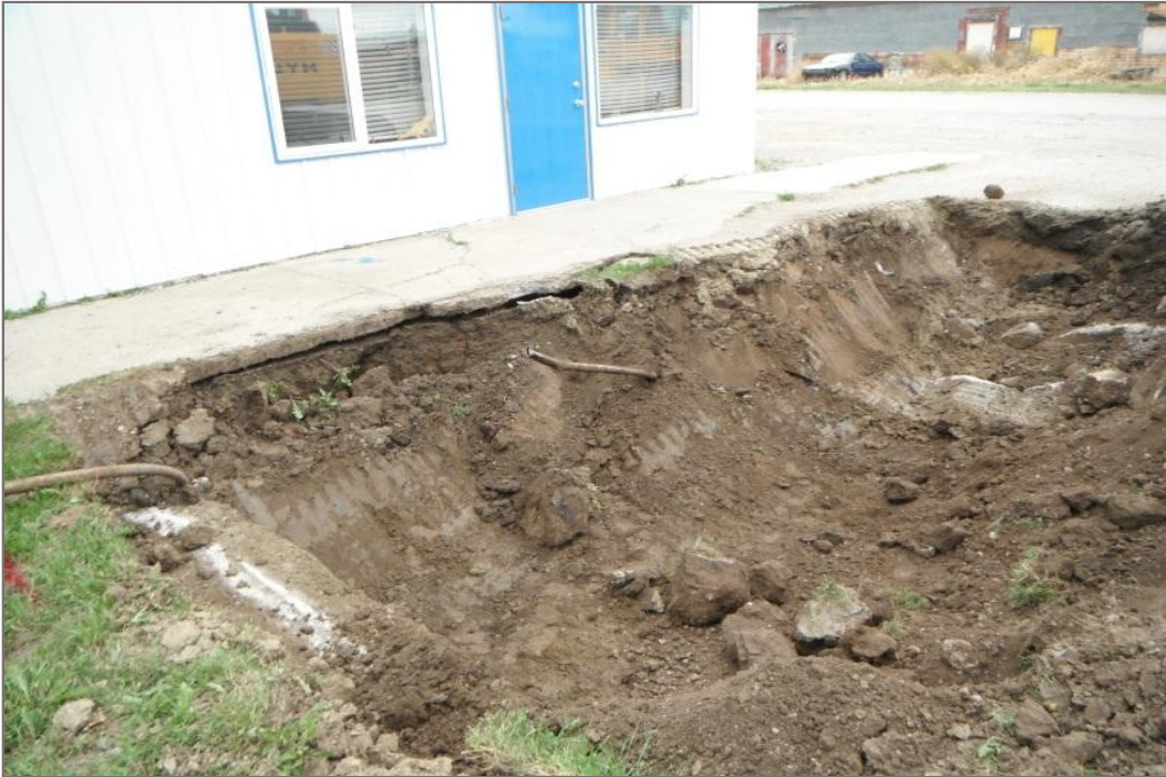
Photo 1: View showing southern boundary of excavation limits and underground piping.
