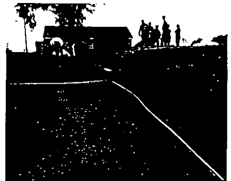
PIPE RUN N.W. CORNER
